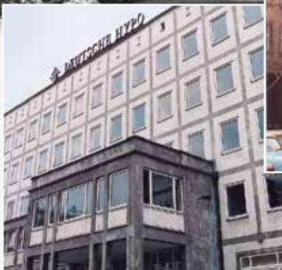
Former front at Georgsplatz 8, Hanover
